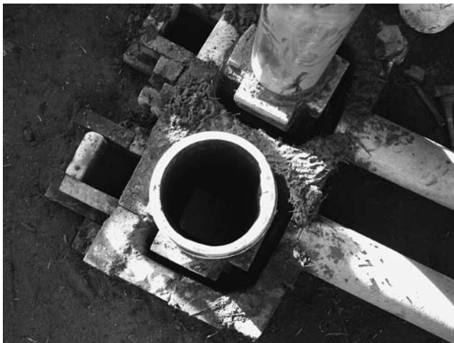
Left: Two Rocket Stoves side-by-side in an experimental session with heat risers of steel instead of brick. The brick fortresses around the burn tunnels form the supports for the heat exchange barrels as well as containment for the gases flowing down the barrels and into the exit flues, at right. The bricks and barrels' bottoms will be sealed from outside with cob.
