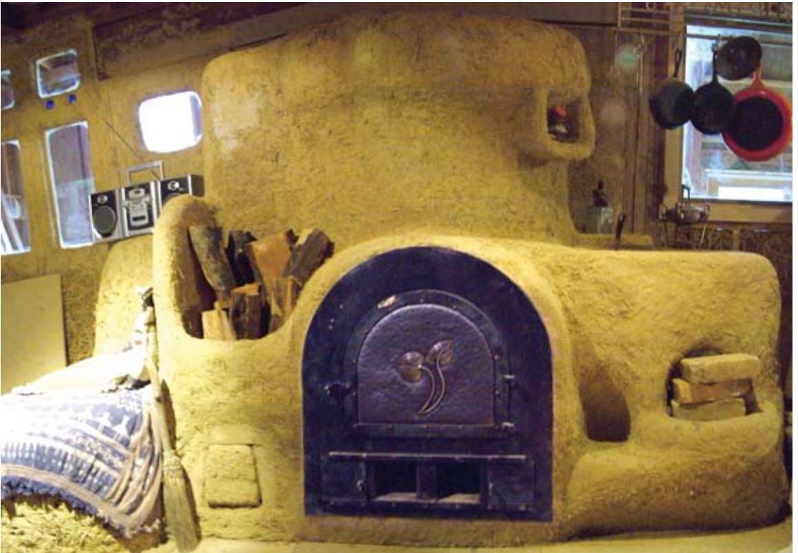
Above: Chris Reinhart's Rocket Stove. Note that the barrel is exposed quite a bit to maximize radiant heat. Below: Kirk Moberg's Rocket Stove with cooking surface on top. There are two cold air intakes below the metal door. The cob bench box keeps firewood dry.
