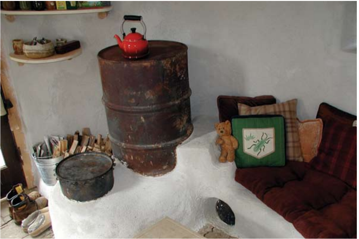
Above: Chris Reinhart's Rocket Stove. Note that the barrel is exposed quite a bit to maximize radiant heat. Below: Kirk Moberg's Rocket Stove with cooking surface on top. There are two cold air intakes below the metal door. The cob bench box keeps firewood dry.
