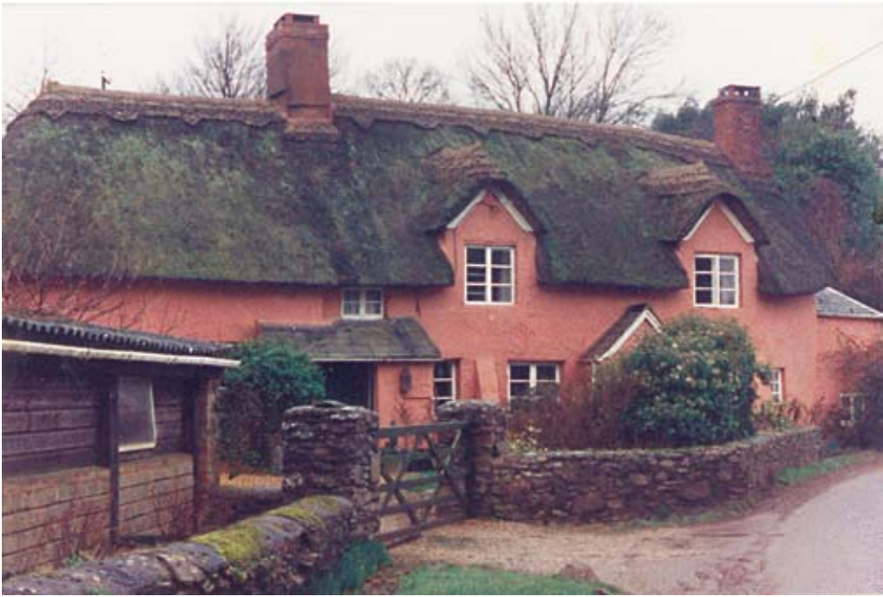
Three examples of cob buildings that have stood for several centuries in southwest England.
